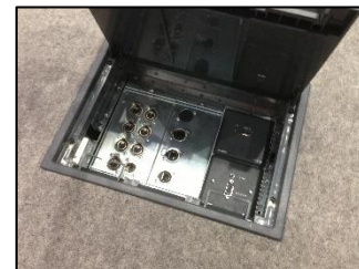
One of the eight platform floor boxes providing discreet connectivity for musicians, microphones, and visual sources
