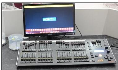
The auditorium also has an effective integrated stage lighting system for highlighting the platform which also works together with the LED ceiling cloud lights. 16 lanterns featuring a mix of coloured spot and floods and controlled via a Zero88 programmable console, allows an array of moods and focal points for musicians and service leaders.
