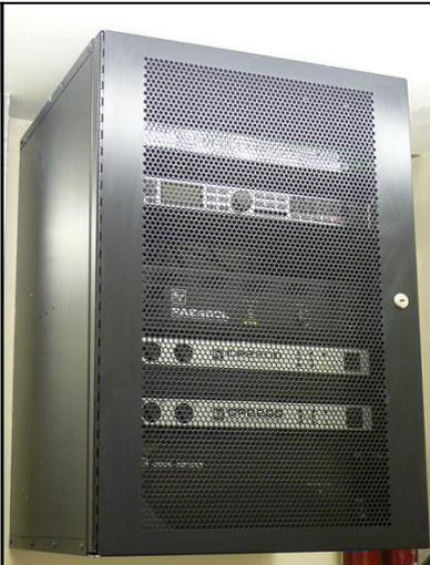
Wall mounted rack for secure housing of all amplifiers and audio control hardware
