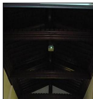
The main projector, an Eiki X71 5500 lumen high contrast LCD model, discreetly mounted within the ceiling wooden beams with full operation controlled via remote touch panel
